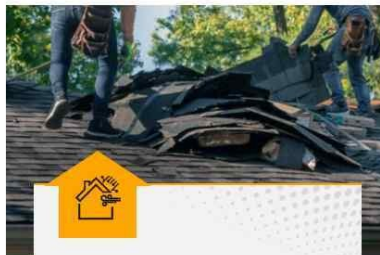
Roof Storm/Wind/Hail Repair
