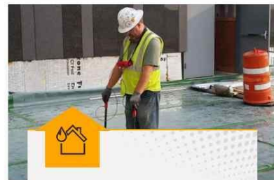
Roof Leak Detection
